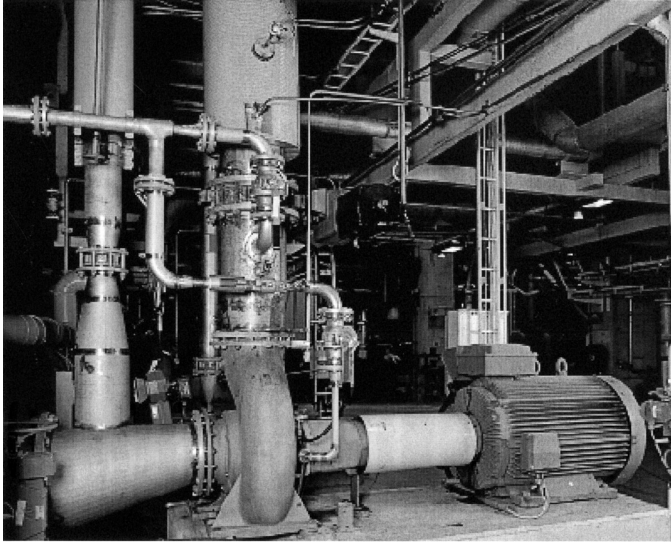
Figure 6.20 In some industrial plant operations, pumping systems account for 25 to 50% of energy use. (Courtesy of, and with joint permission of the Hydraulic Institute, Parsippany, NJ; Europump, Brussels, Belgium; and the U.S. Department of Energy Office of Industrial Technologies, Washington, D.C.)
